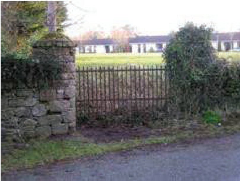
Figure 7.3 – Stone wall, pillars and gate, Naas (note gentle lines and stout pillars)
