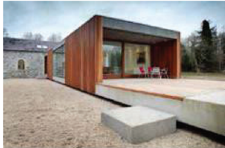
Figure 8.1 – Refurbishment and extension, Ballymahon House (ODOS Architects).
