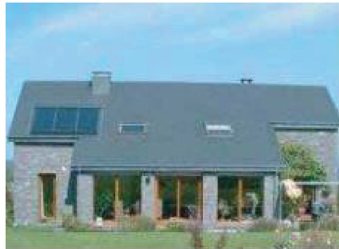
Figure 6.1 – Image of roof solar panel.
