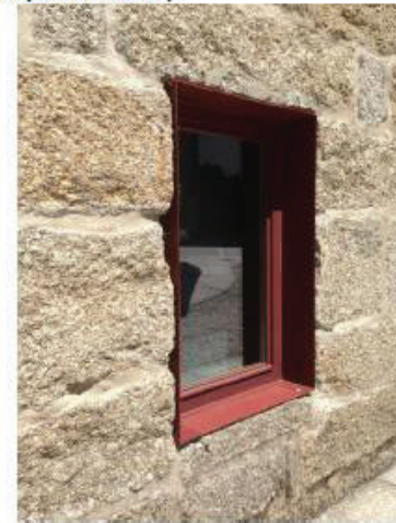
Contemporary window with painted steel reveal.
