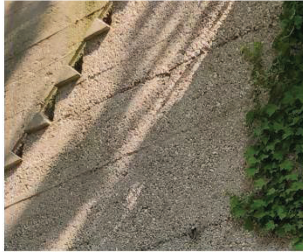
Rough cast concrete.
