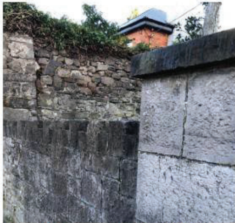
Random rubble, coursed rubble and ashlar stonework.
