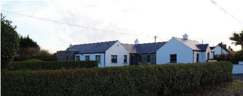
Figure 8.5 – Example of an extension to an old cottage designed to accommodate modern living needs.
