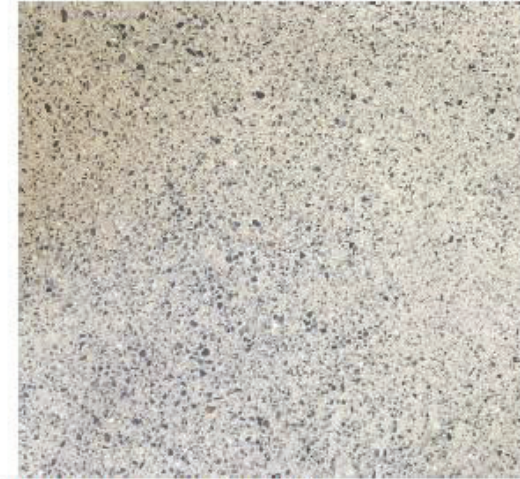
Ground concrete surface finish.
